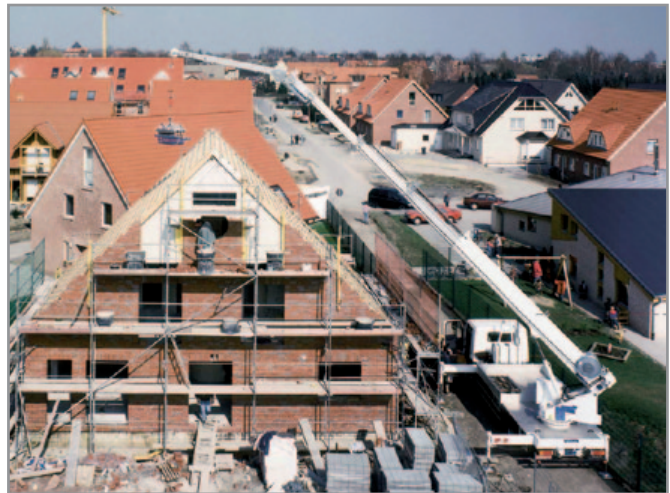
AK 32/4000 PLC reaches the rear side of the roof without any problem
