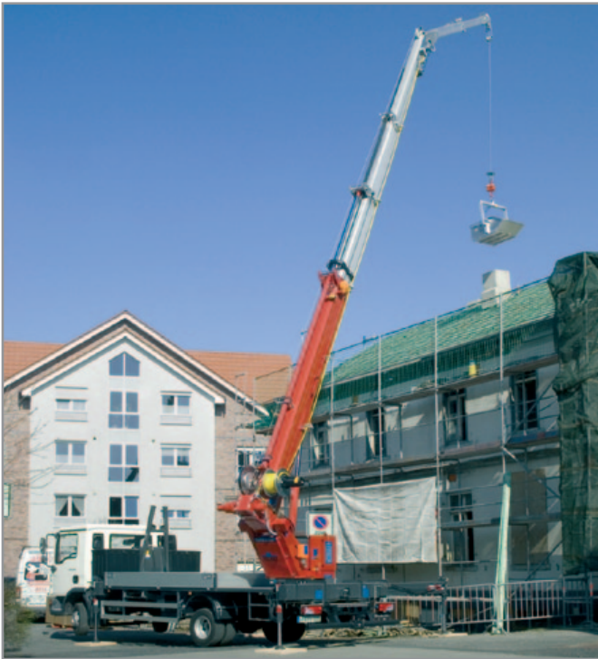
Truck Crane AK 32/1500 PLC
